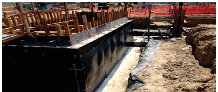
Above: Installation of Membrane Protection Board
