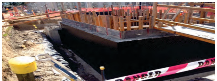
Above: Final Coat of Duroproof BLW (Cured)
